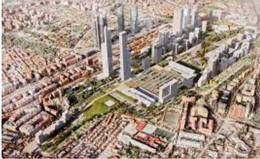
Figure 5 - Madrid's Charmartin HSR Station serves northern HSR lines and is being connected to Atocha Main Rail station via a new rail tunnel.
